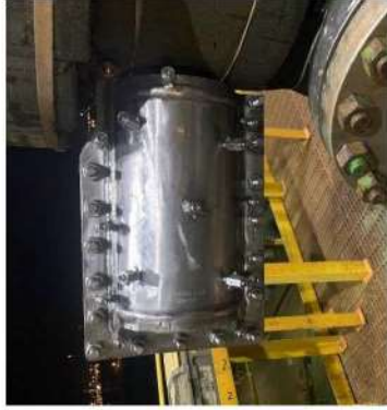
Figure 1. A temporary pipe clamp over a valve that had been leaking
